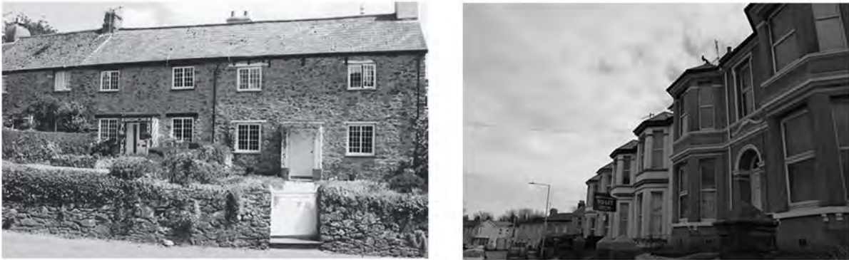
Figure 46 The uniform treatment of the boundaries make a significant contribution to the character of the street.
