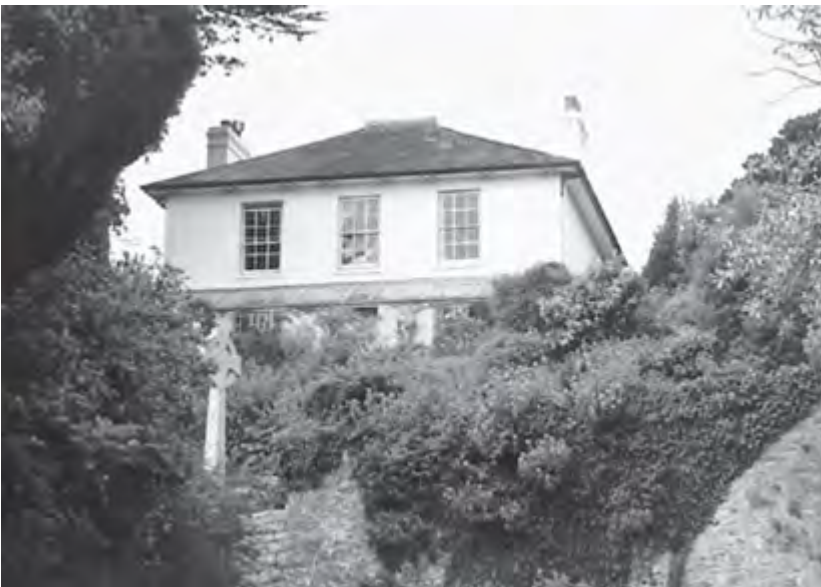
Figure 56 The 'polite' style of this 19th century house derives from the formality of its architectural treatment which creates a dignified and refined appearance
